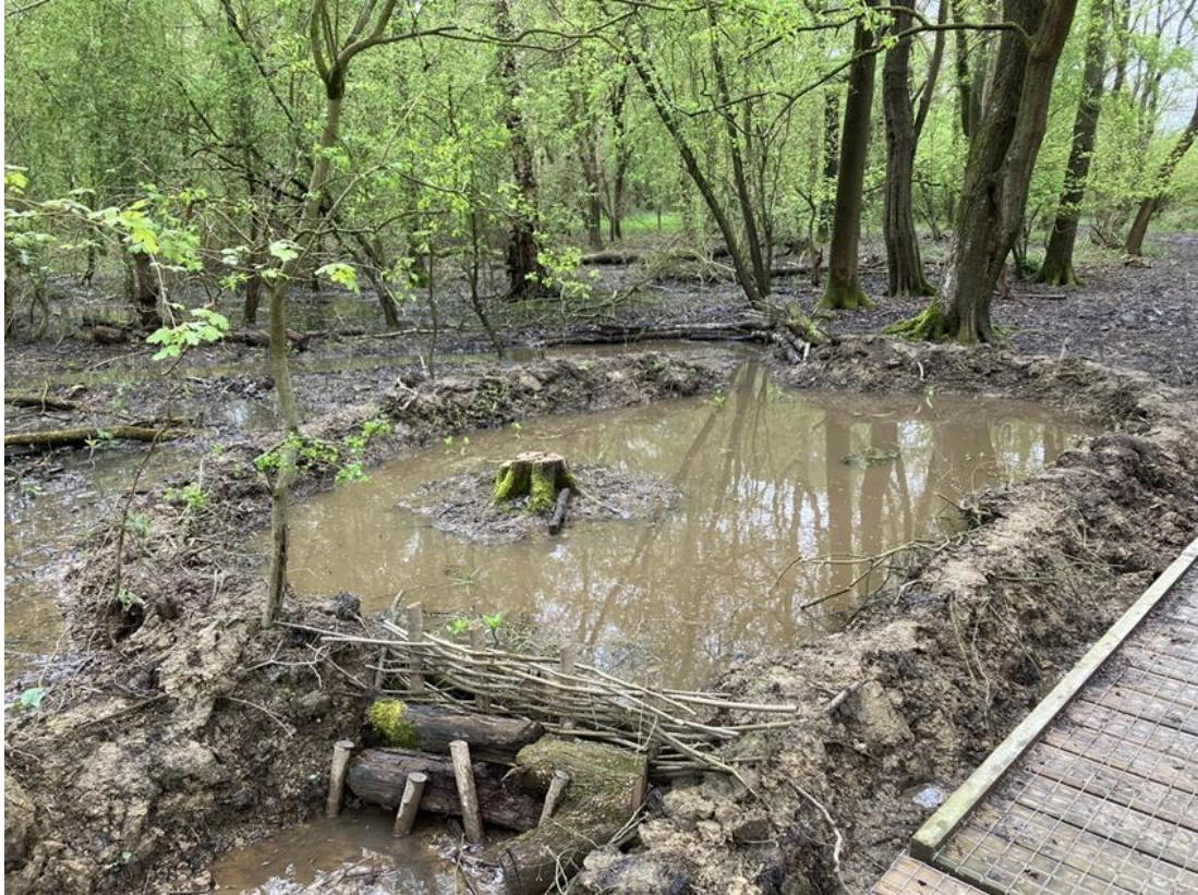
Photo 4. A recently constructed shallow scrape fed by woodland ditches with leaky dams adjacent to the board walk. (late April 2023)
